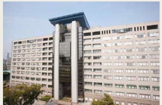
▲入院棟 Ward (University Hospital)
